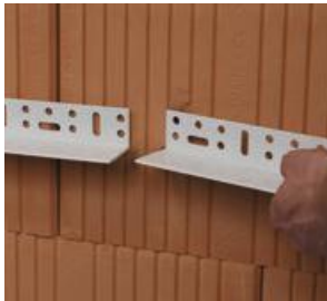
Attach angle rail
