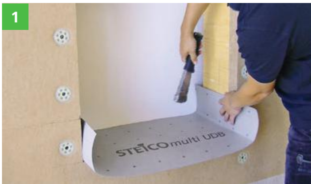
Attachment of STEICOmulti UDB (diffusion-open membrane) as temporary weather protection until window installation.
