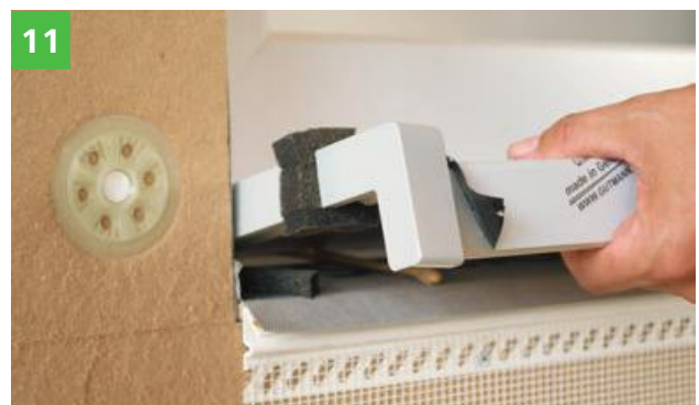
Installation of windowsill. TIP: The rear sheet metal interlocking is located in the matching window groove, the front one has a distance of \geq 3 cm to the render facade Tip: Storing Compriband strips in the cool box prevents them from expanding too quickly.
