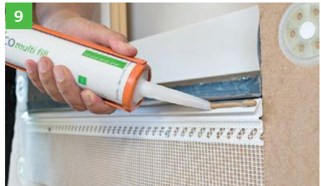
The protruding flap of the laminated underlay is glued to the drip edge of the parapet profile using STEICOmulti fill.
