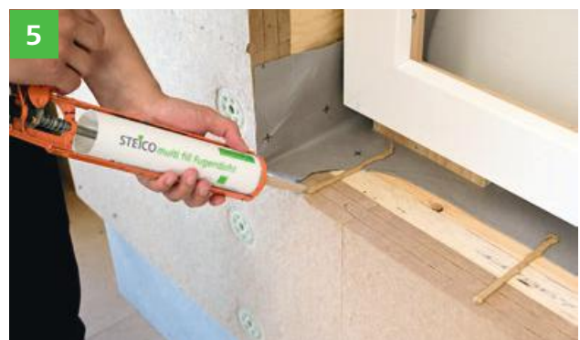
STEICOmulti fill adhesive beads are used to secure the insulation wedge against lifting off, e \leq 30 cm.
