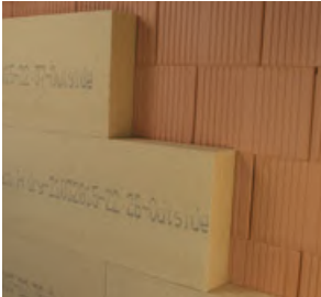
Installation of small-format square edge boards
