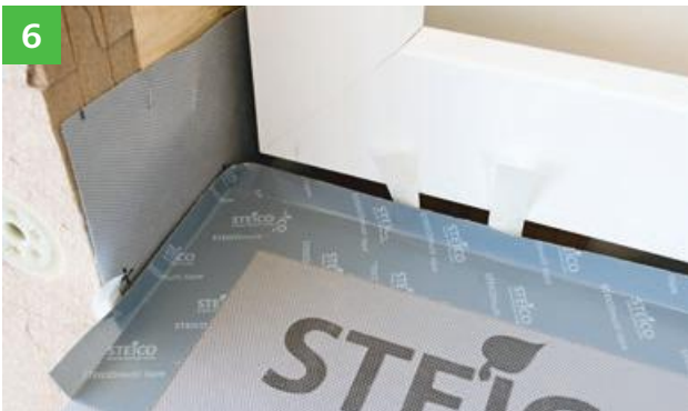
Installation of the STEICOfix insulation wedge. TIP: Fold back release paper, it can be removed more easily later.
