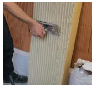
Glue the insulation board to a flat surface with full-surface bonding
