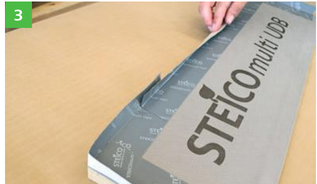
The STEICOmulti tape F adhesive strips are then attached to the insulation wedge in such a way that a three-sided „trough“ is formed.
