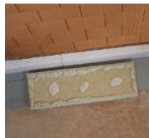
Adhesion of insulation boards on uneven surfaces using the point and bead method
